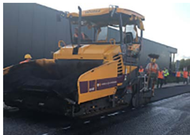
Constructing a lignin asphalt test strip
