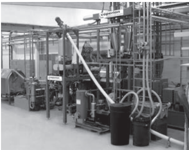
Compounding plant for the production of WPC wood plastic composites
